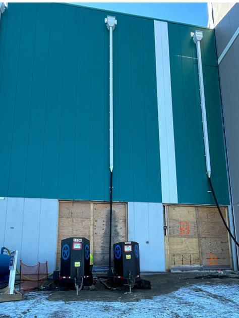
**Delivery, Safety and Setup** – Within one week of the demonstration of one Jet Heater, twenty nine (29) Jet Heaters surrounded the building. Following safety training and jobsite initiation, a team of technicians from REIC were on site to perform setup and startup of the units, with no reported issues. All units sat at the exterior of the building, delivering heating through temporary openings and running hot air through ducting to various points throughout the interior.
