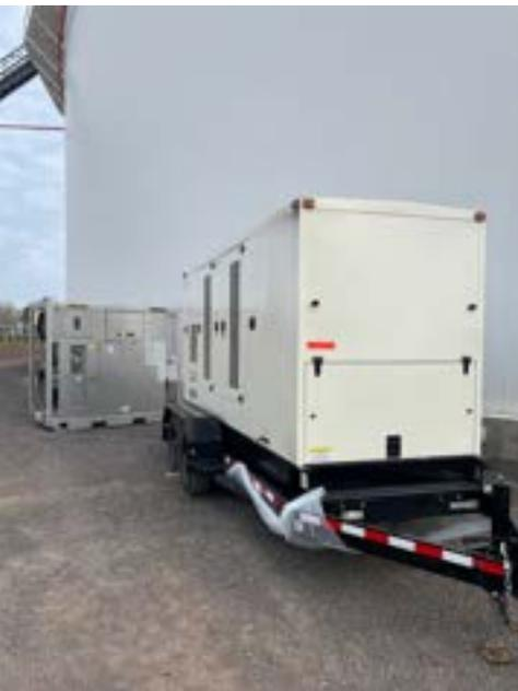
**Temporary Installation and Delivery** - In order to both maintain steel temperatures and help prevent flash rusting, both heating and dehumidifiers were brought to the tank project. Two (2) 60kW in-line heaters were paired with a 5000cfm dehumidifier per heater, working together to maintain a consistent temperature and dew point inside the tank.
